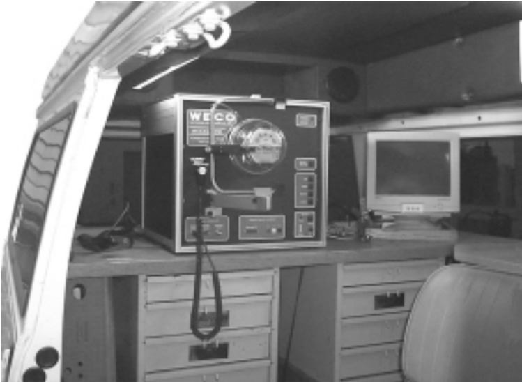
Figure 14-17. Mobile Meter Testing Facility.
