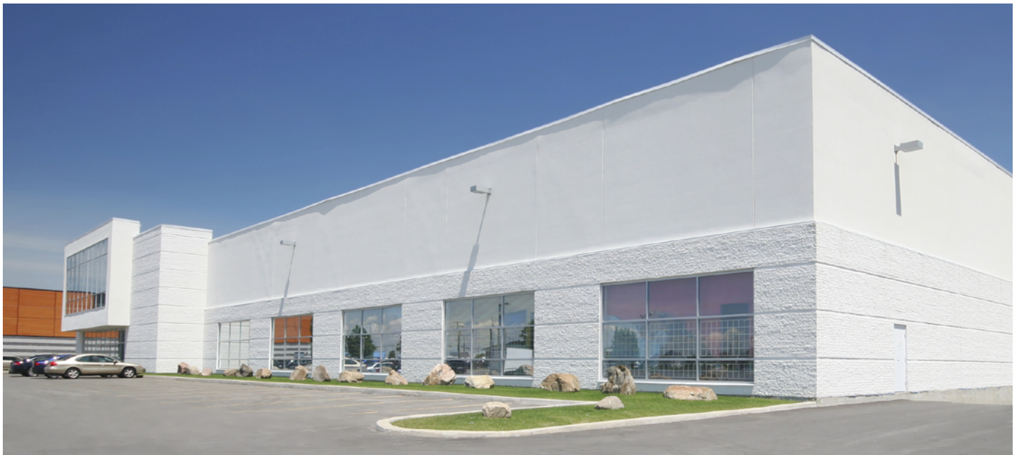
Commercial building with 200A nominal service, 277V.
